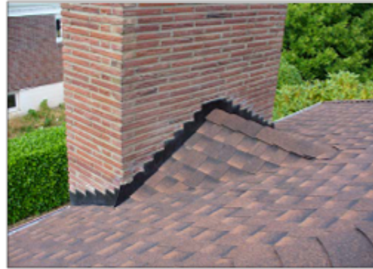
Cricket or saddle at chimney.
