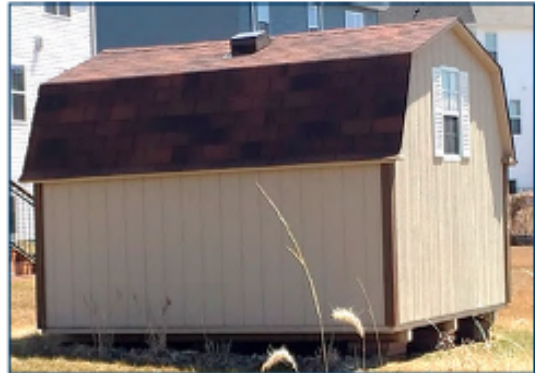
A manufactured storage shed with wood skids.
